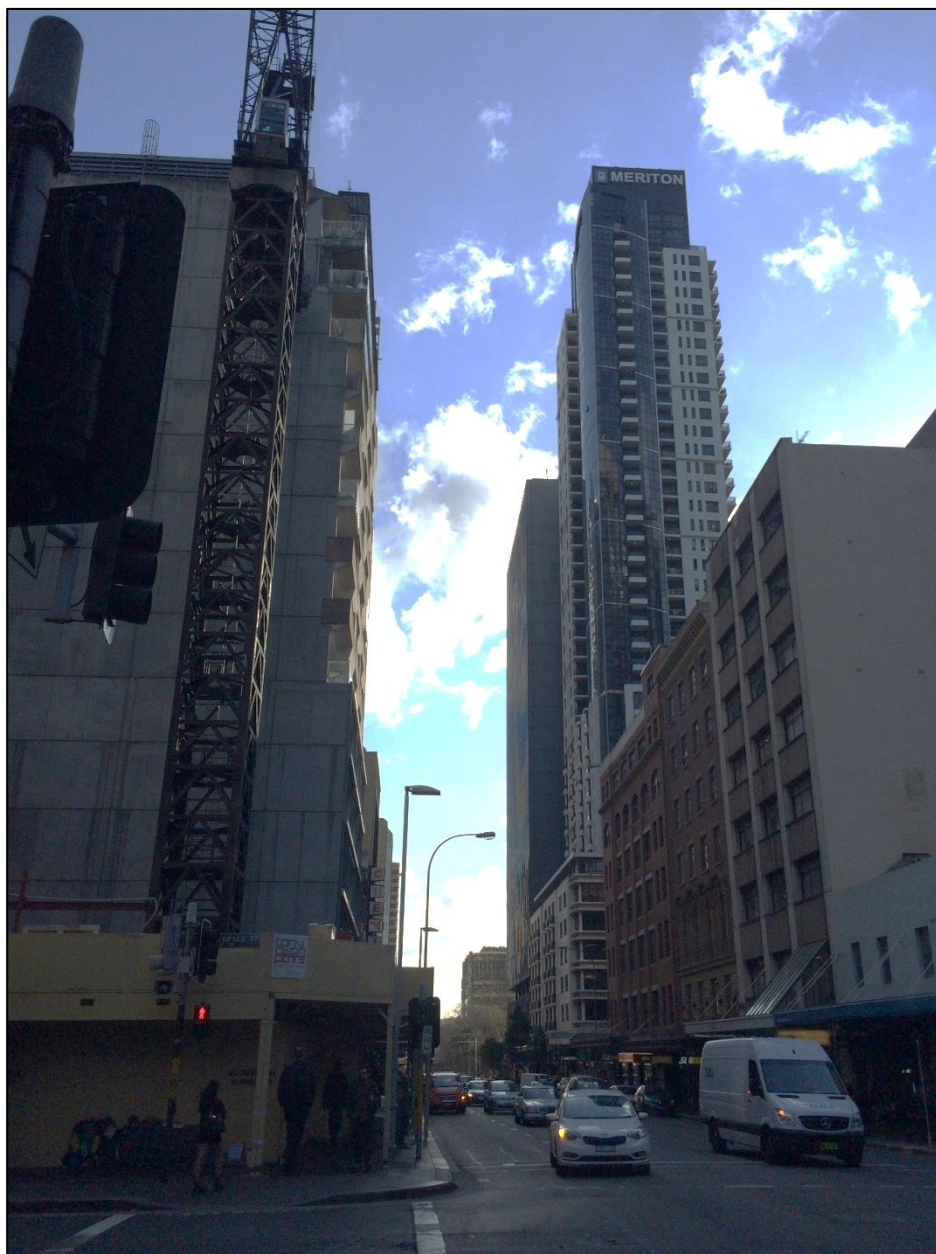
Figure 5: View of development surrounding the site looking west along Bathurst Street, including construction site (at 141-149 Bathurst Street) to the south of the site
